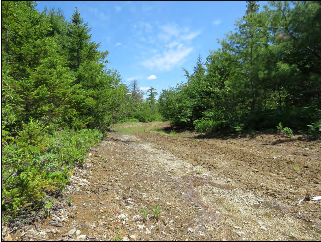
PLATE 15: Example of roads connecting to Seloam Lake Road. Facing west; July 4, 2018.
