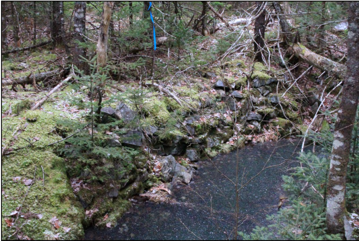
PLATE 29: Site 7 as seen during 2018 reconnaissance showing tiered stone channel leading from crusher. Facing north; December 8, 2018.
